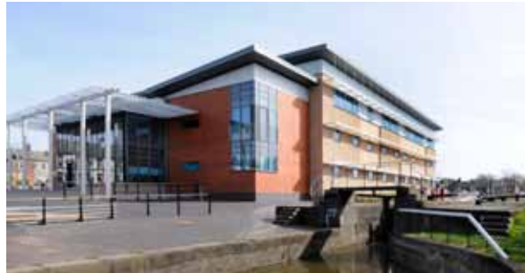
Figure 1.8: Contemporary use of traditional materials at South Shelton Health Centre - buff brick, staffordshire blue brick and terracotta cladding
