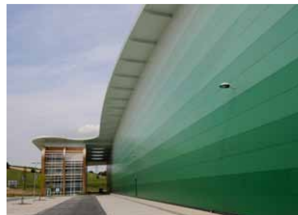
Figure 8.7: Blue Planet, large scale carbon positive industrial development that uses a sculptural form and a gradation in colour on its elevations to make sure it sits well in its surroundings. All of its energy and heat comes from renewable sources and its drainage is sustainable, with rainwater harvesting and controlling of surface water run-off on site, using a series of ponds which have been landscaped to enhance local ecology and to create areas with public access
