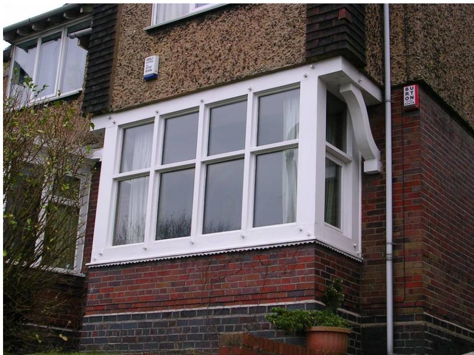
**FIGURE 10:** 13 Victoria Park Road – wet dash render above smooth red brickwork
