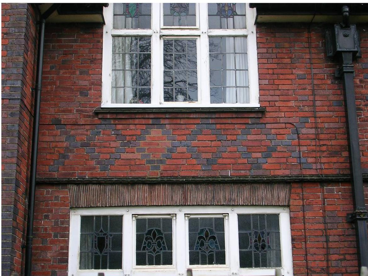
**FIGURE 9:** *Diaper brickwork and tile window heads.*
