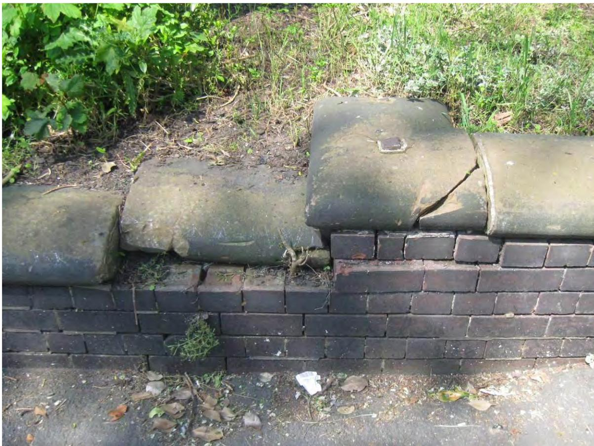
**Fig 27:** Stone copers to the boundary walls have been dislodged, with damage to brickwork
