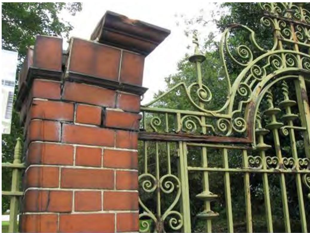
**Fig 38:** Gatepost in poor condition
