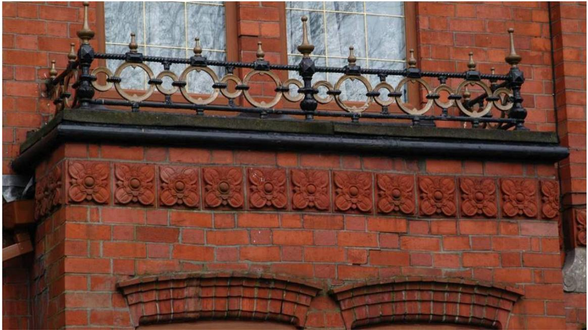
**FIGURE 7:** *Façade finishes: Flemish bond brickwork with moulded brickwork frieze panels.*
