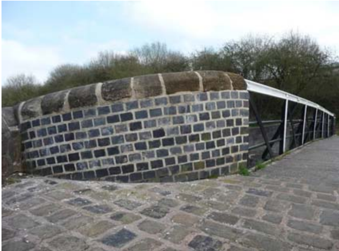
Fig. 5: Header bond and stone copers to brickwork in Bridge 130, with traditionally designed stone setts and metal railings
