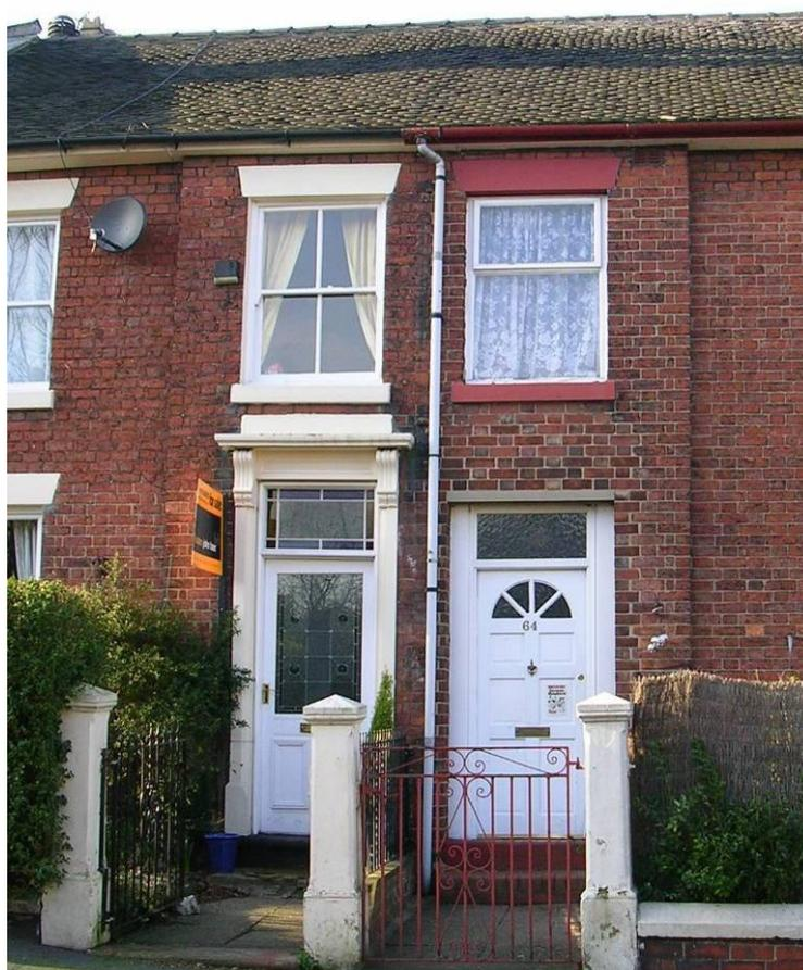
**FIGURE 21:** *Harmful modifications. Removal of timber detailing, sash windows and timber doors and replacement with inappropriate uPVC*
