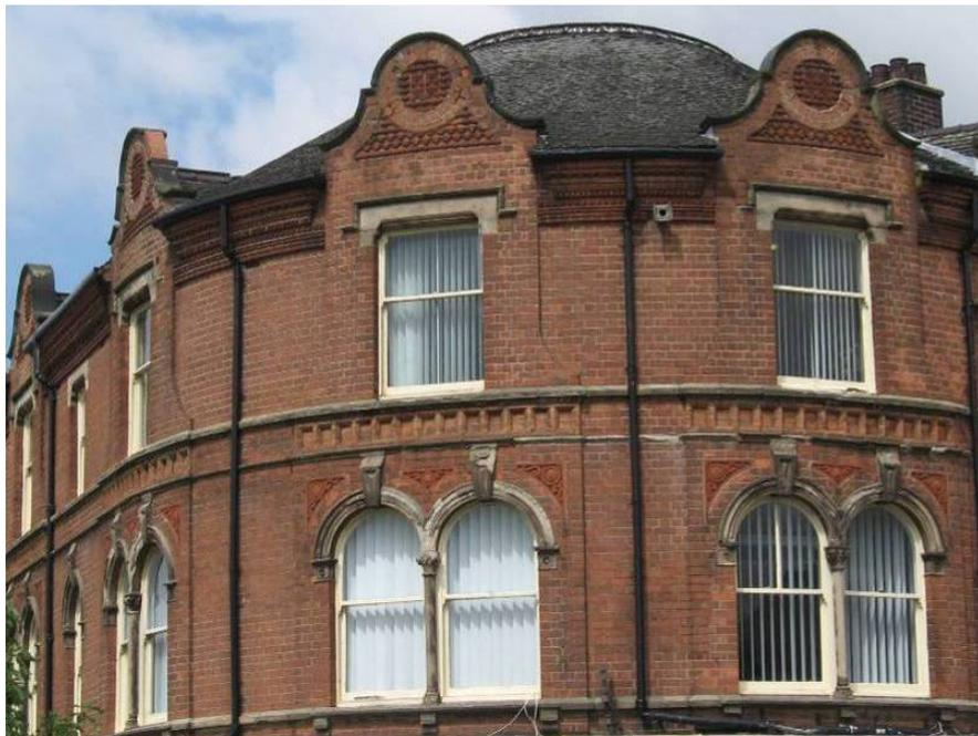
**FIGURE 20:** Brick detailing and stone window surrounds
