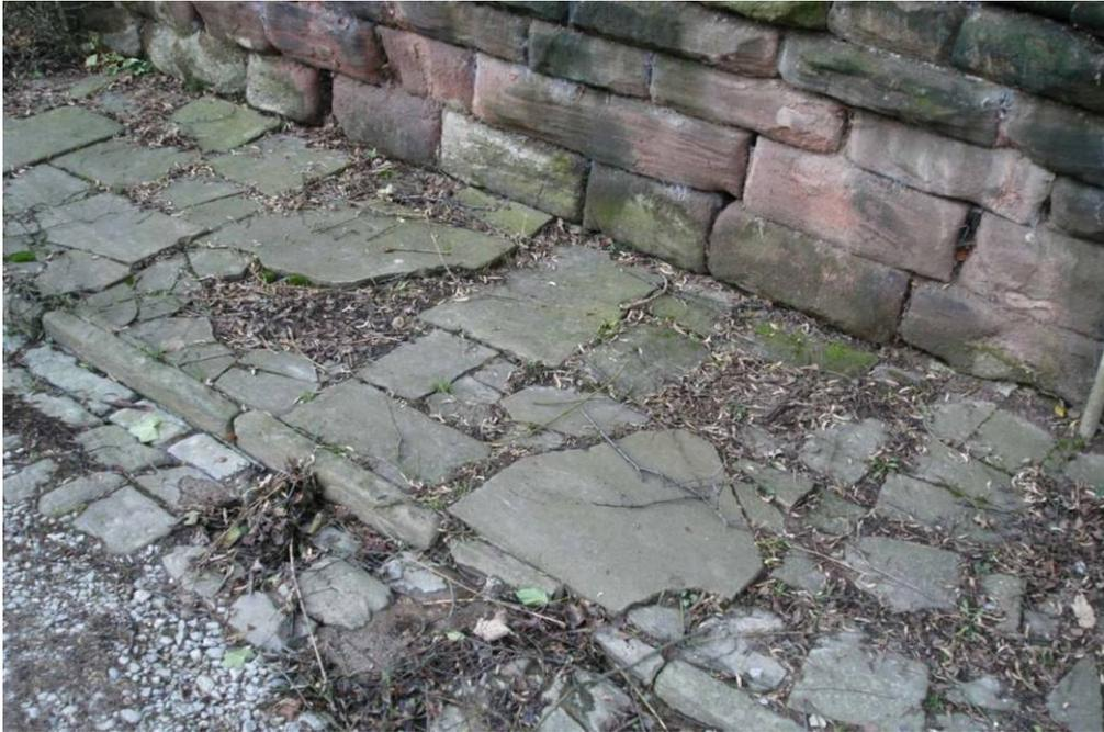
**FIGURE 8:** *Sandstone wall and york stone pavements adjacent to no. 9*
