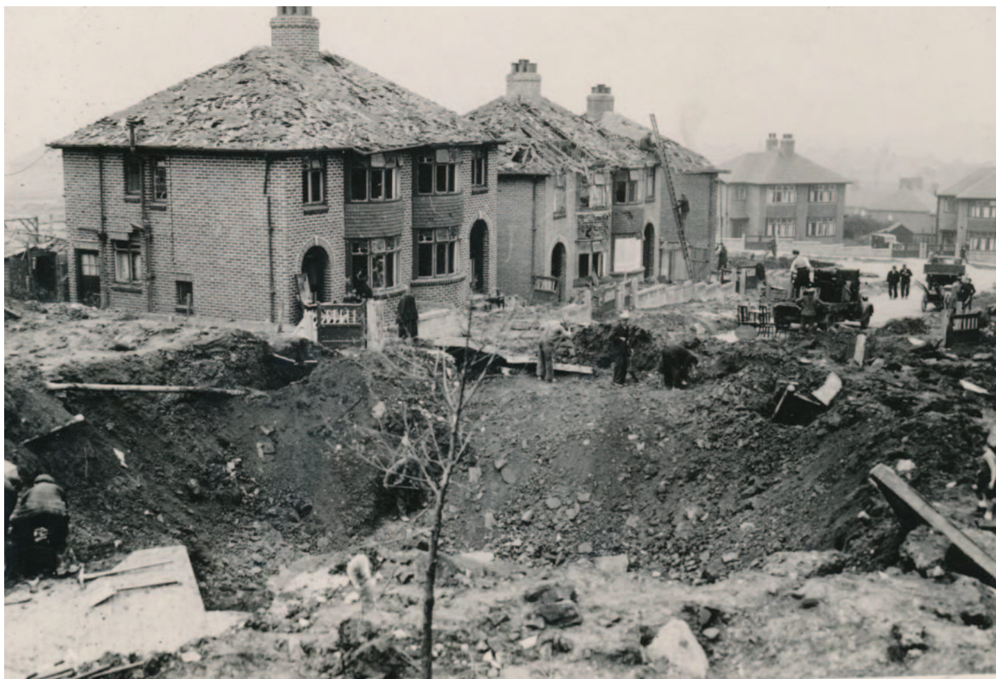
Figure 5: Bomb damage at Taylor Avenue, Maybank, June 1941, Image courtesy of The Potteries Museum & Art Gallery, Stoke-on-Trent
