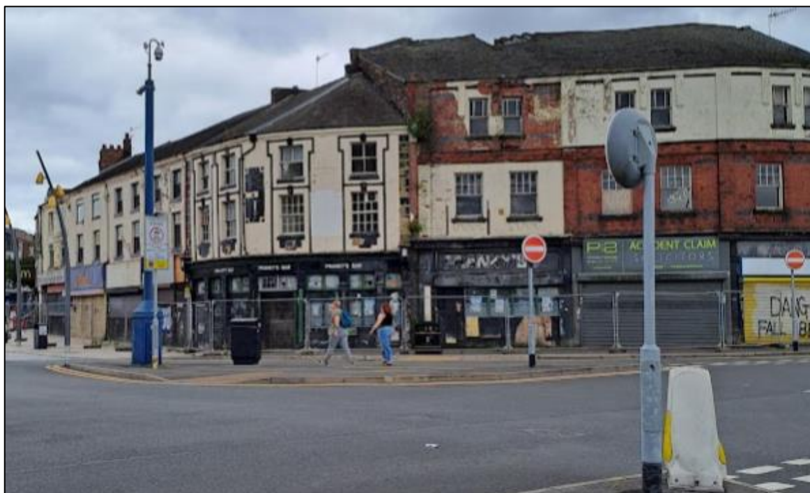
Figure 18: Vacant Units, Parliament Row/ Old Hall Street
