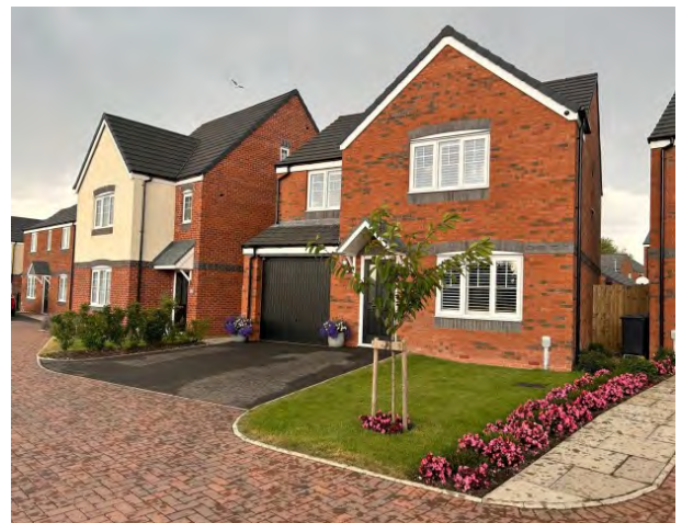
Picture 2 11320 - Land to the west of Caverswall Lane
