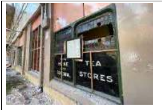
Photo 22 - Etched glass internal windows damaged.
