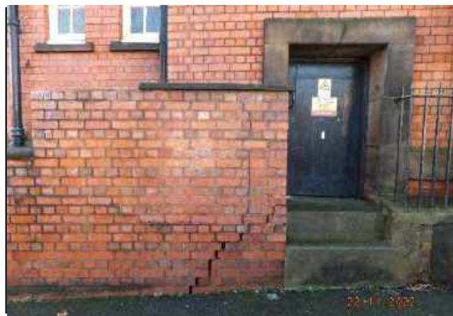
Photo 58 - Stepped cracking to freestanding wall on Price Street.
