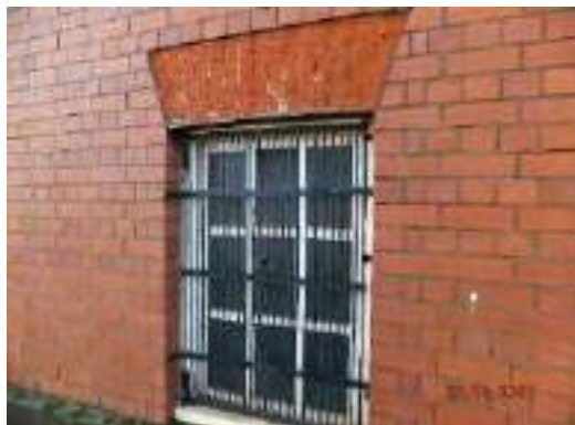
Photo 98 - window to East elevation along Price Street - mock stone finish to brick flat arch has been lost.
