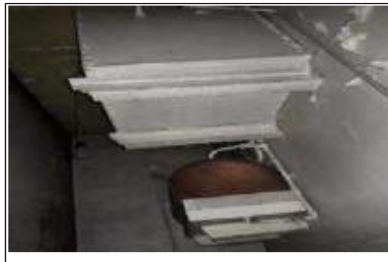
Photo 38 - Cold water storage tank and hot water cylinder
