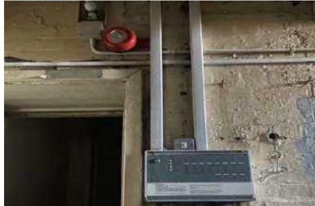
Photo 8 - Redundant fire alarm panel
