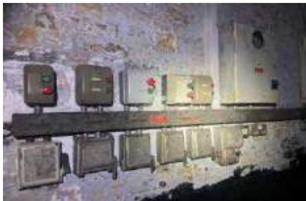
Photo 2 - Electrical switchgear and basic heating control panel
