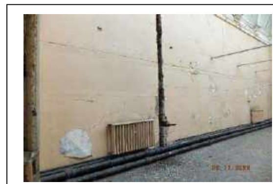
Photo 24 - exposed internal downpipe to RF.23.
