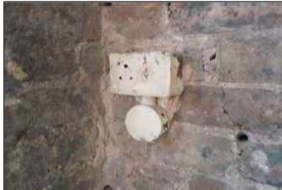
Photo 44 - Socket outlet 50+ years and defective
