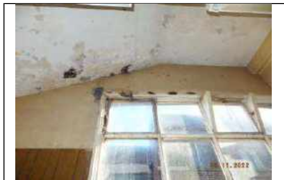
Photo 17 - RF.36 (student room). Water ingress and associated damage.
