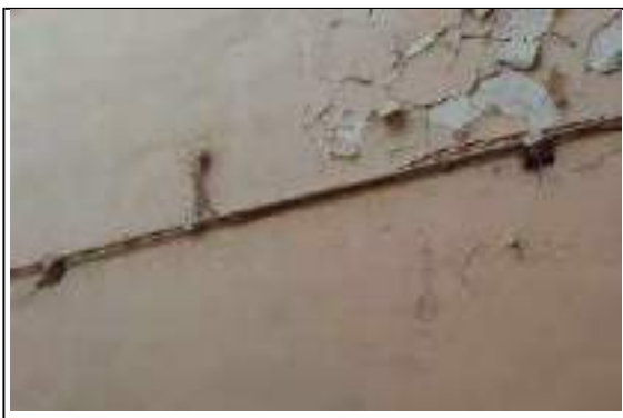
Photo 49 - Single core cables not fully intact.
