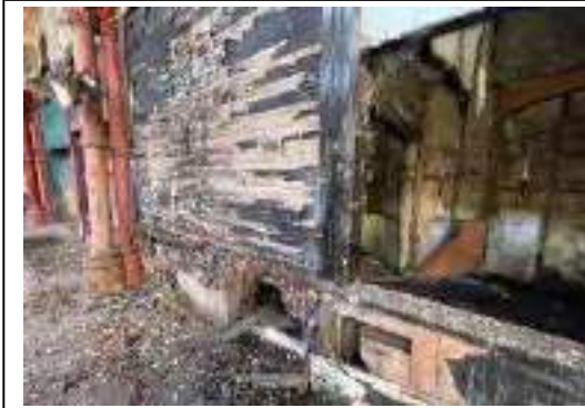
Photo 20 - Timber decay and overall disrepair of another unit.
