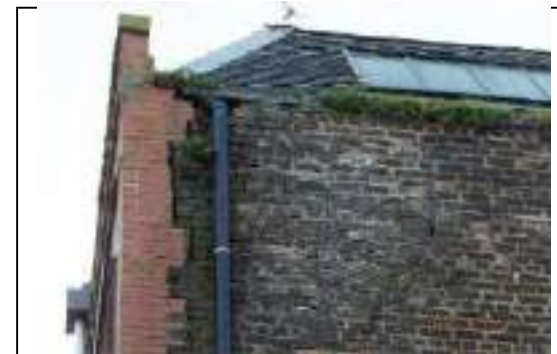
Photo 6 - Brick junction opening up between East façade at parapet level and North elevation. Rainwater disposal system blocked by vegetation.
