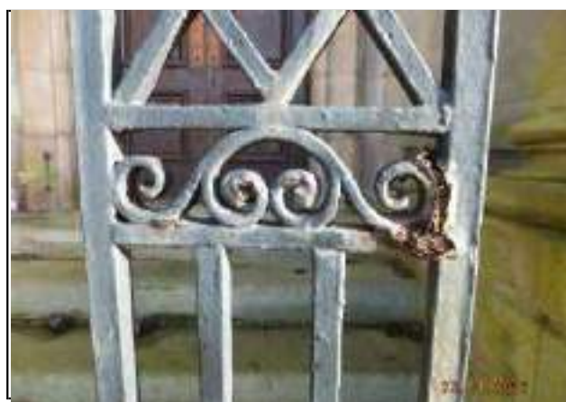
Photo 65 - Corrosion damage to railings.
