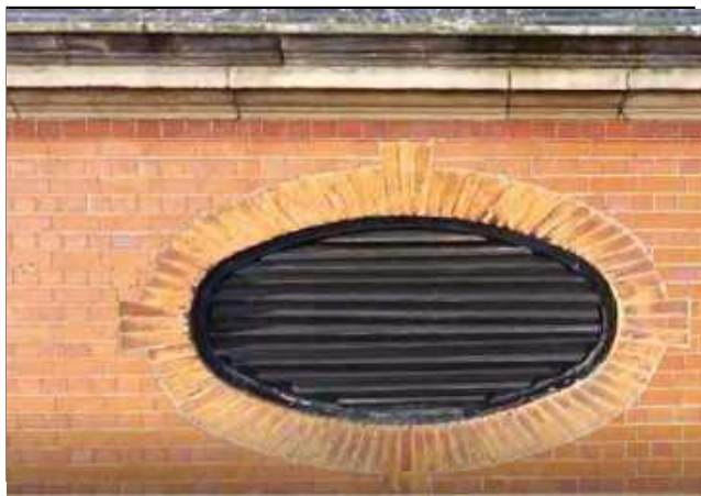
Photo 88 - Spalling to brick surround at high level.
