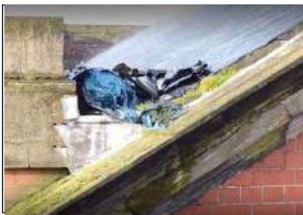
Photo 86 - Debris blocking rainwater discharge on roof.
