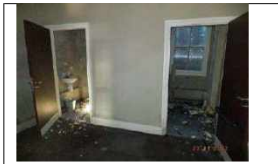
Photo 14 - RG.19 Damage to sanitary facilities due to leak. Dry rot observed to RHS skirting level.
