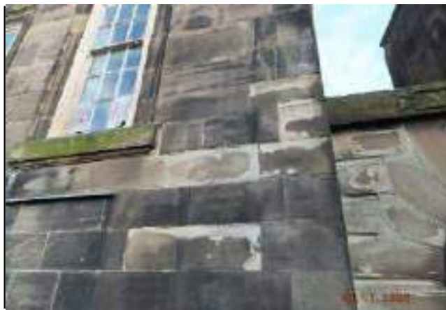
Photo 70 - Example stone deterioration due to staining and cementitious pointing.
