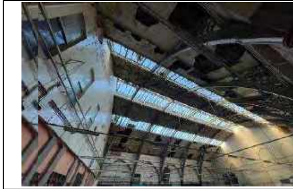
Photo 8 - Overview of the Market hall roof, cast iron, glass and lath and plaster, in poor condition.
