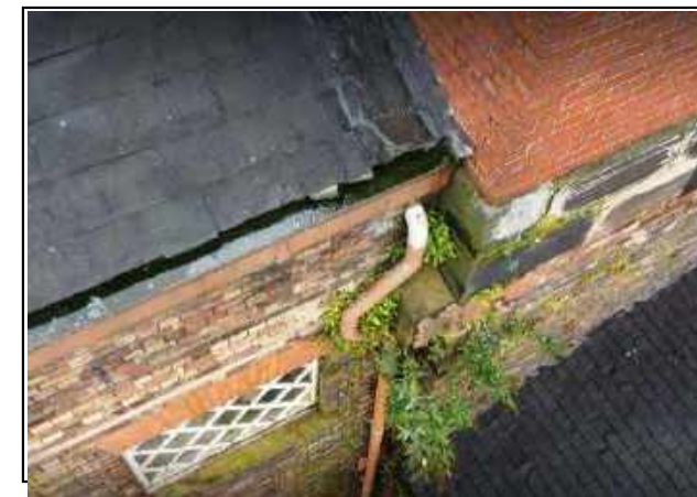
Photo 84 - Poor detail and disrepair to downpipe/ outlet in central courtyard. Note, photo taken from 2021 survey not current.
