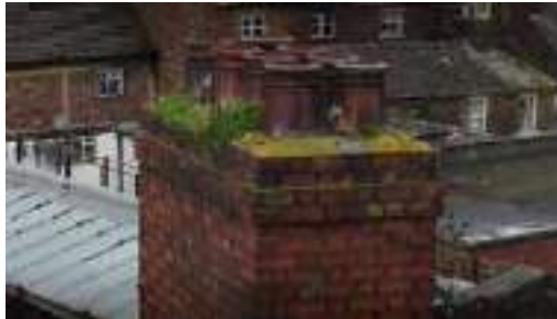
Photo 46 - Vegetation growth to the chimney pots.
