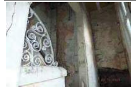
Photo 33 - Root growth observed down internal first floor wall of rear stairwell.
