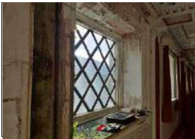
Photo 74 - Example cast iron lattice fixed window.
