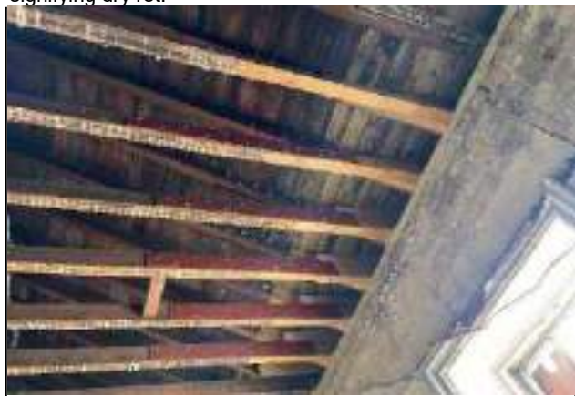
Photo 40 - Example of the timber splicing to the roof trusses of the first floor within the office space.
