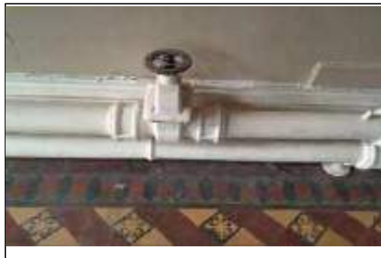
Photo 35 - Heating pipework gate valve
