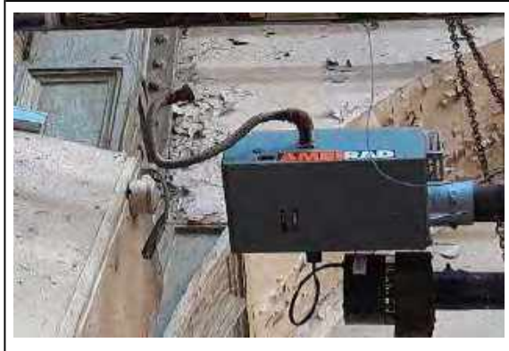
Photo 31 - Radiant tube gas burner disconnected from gas supply.
