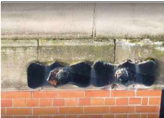
Photo 89 - Example lateral restraint plates.
