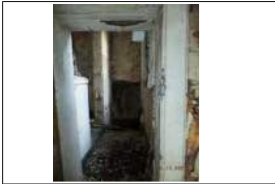
Photo 31 - View through to stairwell from RF.26 (no further safe access). Decayed & failed lintel, extensive damage to woodwork and plaster. Pigeons freely using the space.
