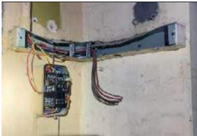
Photo 19 - Existing redundant wiring installation and fusegear
