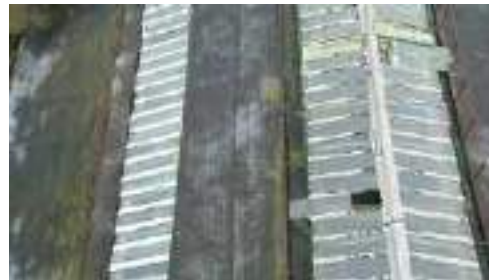
Photo 41 - Slipped glass panels.
