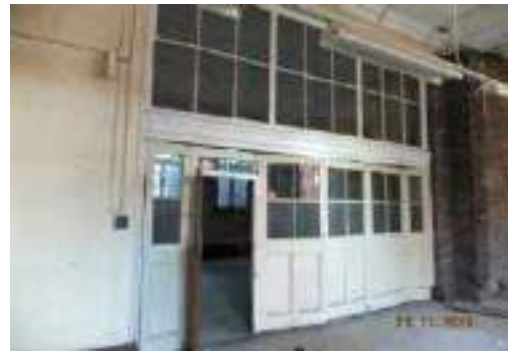
Photo 29 - Folding shutter partition between RF.25 & RF.26 workshops. Note missing/ damaged brickwork to structural pillar on RHS.
