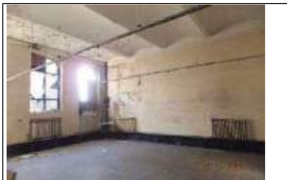
Photo 16 - RF.40 (meeting room). Jack arches visible to second floor.
