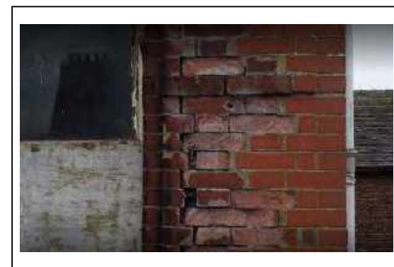
Photo 54 - Displaced brickwork due to previous shrub growth in wall (drone footage).
