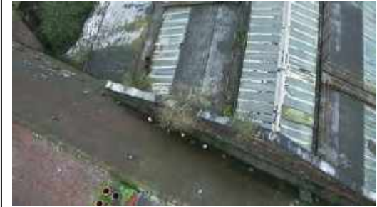
Photo 45 - Vegetation growth to the junction of roofing.
