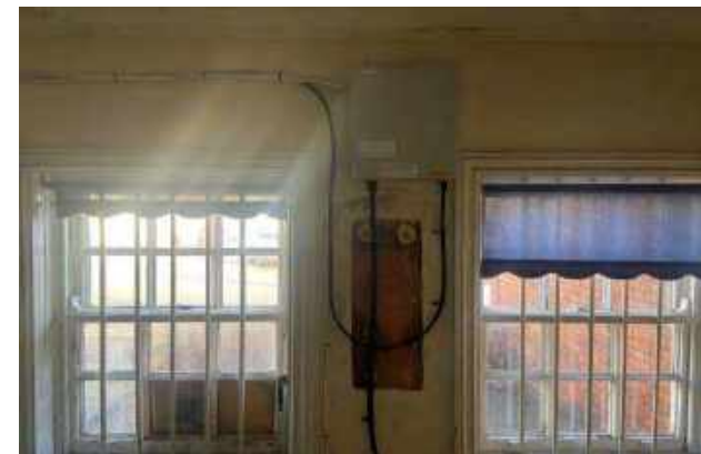
Photo 6 - Temporary LV distribution board
