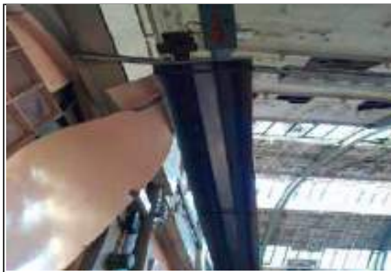
Photo 34 - Gas fired radiant tube heater
