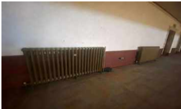
Photo 10 - Typical auditorium area steel column radiator
