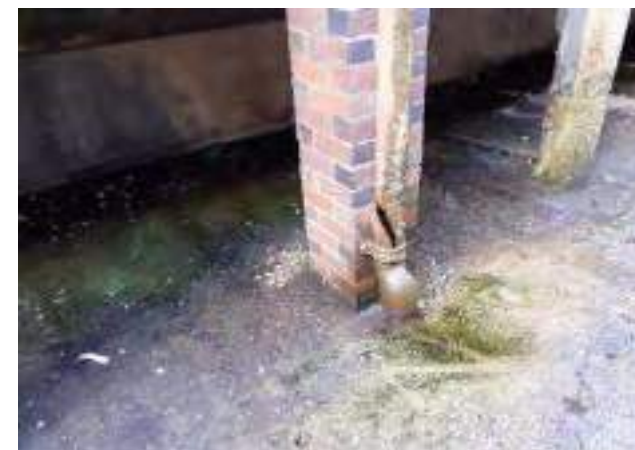
Photo 75 - Inner courtyard ponding and broken downpipe.
