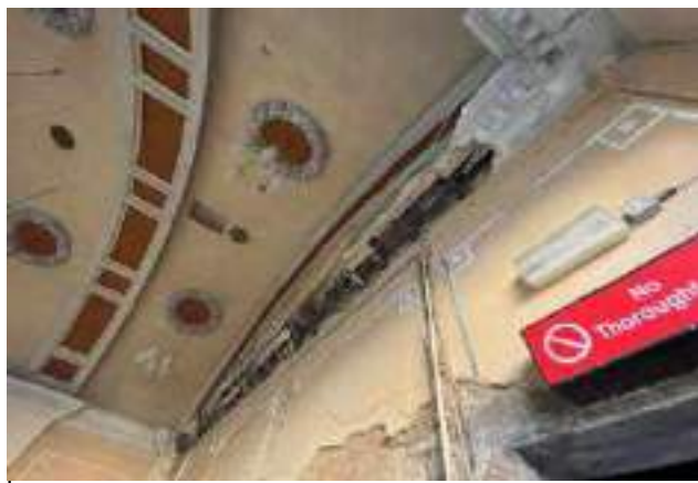
Photo 43 - Ceiling to the small hall where the ornamental plasterwork has fallen.
