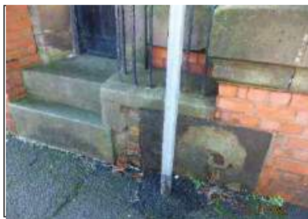
Photo 59 - Damaged cement finish.
