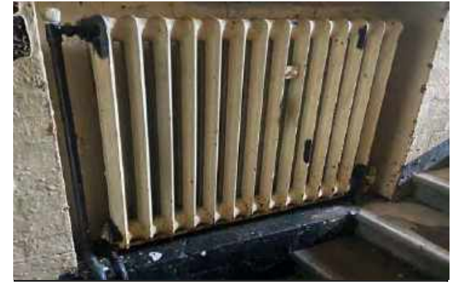
Photo 9 - Typical corridor area steel column radiator
