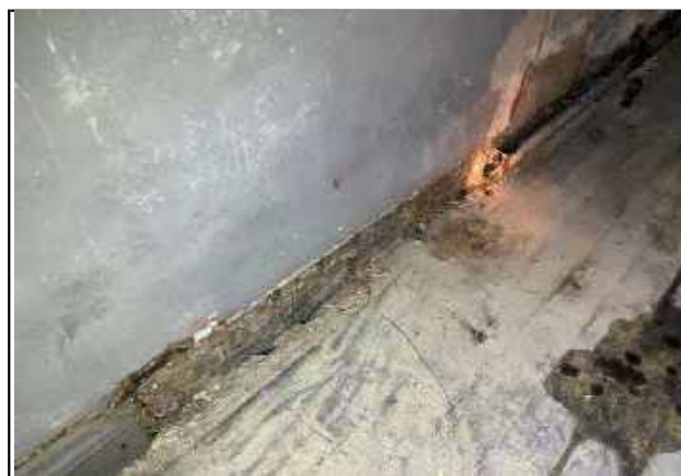
Photo 29 - Dry rot to the timber skirting board in the gallery loft.
