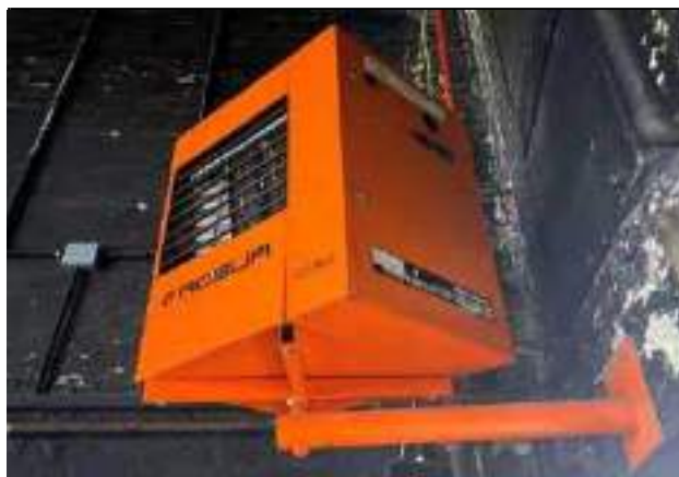
Photo 26 - Gas fired space heater in stage area
