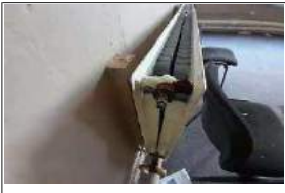
Photo 37 - Radiator showing signs of corrosion
