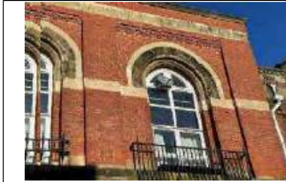
Photo 2 - Second floor windows, and stonework window surrounds showing signs of erosion.
