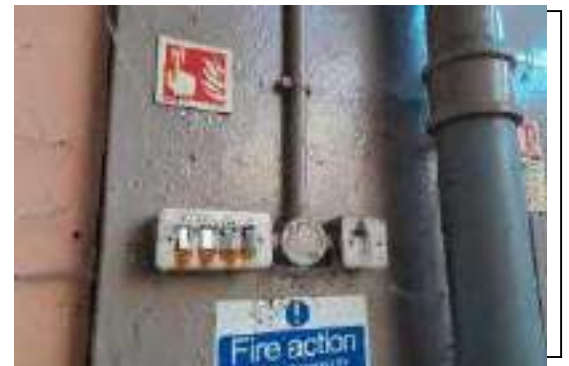
Photo 30 - Corroded light switches
