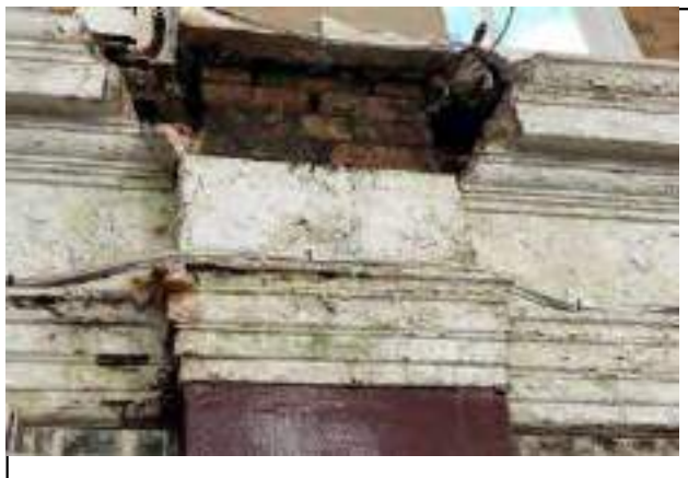
Photo 49 - Exposed brickwork to the internal walls of the ground floor corridor where plaster has fallen.
