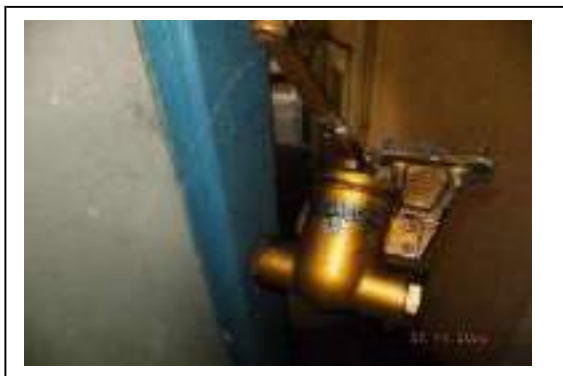
Photo 19 - Example of early 20th Century door closers observed in the building. These should be retained where possible and overhauled by a specialist.
