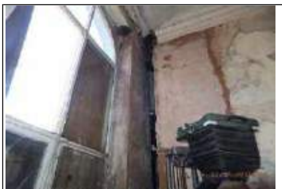
Photo 22 - Plaster & brickwork has been broken out to allow access to internal downpipe in RF.40.
