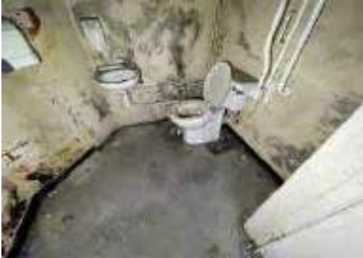
Photo 13 - Significant mould and defective finishes observed to the accessible toilet.
