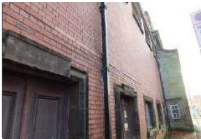
Photo 76 - Displaced lateral brickwork.
