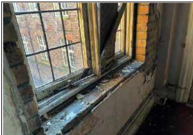
Photo 38 - Exposed brickwork to the window cill of the small hall on the first floor.
