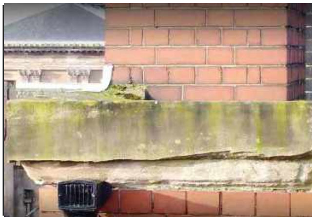
Photo 81 - Deteriorating stone to parapet along Price Street.
