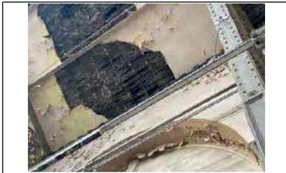
Photo 10 - Lath and plaster ceiling suffering significant decay.
