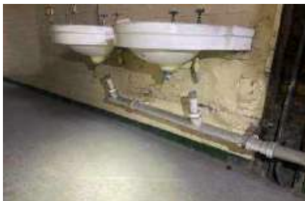
Photo 17 - Existing open-ended waste pipework, and existing lead domestic hot and cold water pipework
