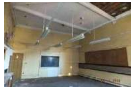
Photo 27 - RF.24 (workshop). Water damage to lath & plaster shown top left, assumed to be historic leak pre-2016 roof repair.
