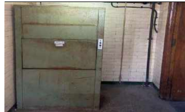
Photo 15 - Redundant dumbwaiter (2 of 2)
