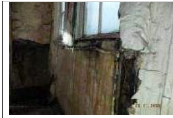
Photo 32 - Severe decay to woodwork and wall finishes beyond RF.26.
