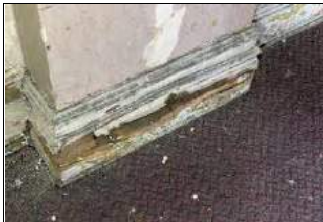
Photo 37 - Cuboidal cracking to the corridor skirting board signifying dry rot.
