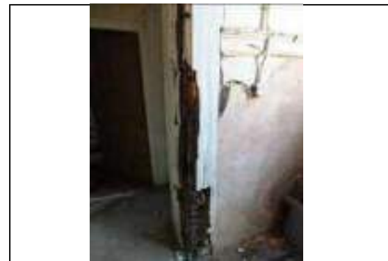
Photo 21 - Architrave destroyed by dry rot in RF.40.
