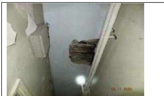
Photo 10 - Example of damaged lath & plaster ceiling to RG.12
