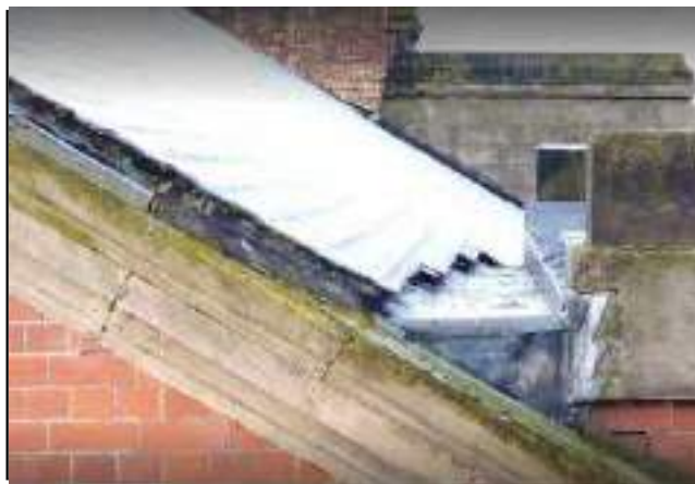
Photo 85 - Example lead lined gutter in satisfactory condition.
