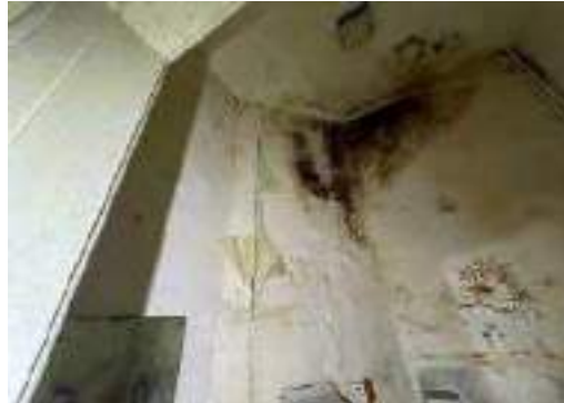
Photo 14 - Mould to the ceiling and walls of the toilets.
