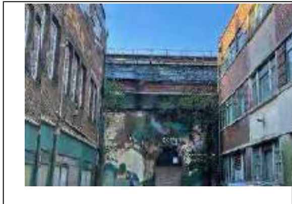
Photo 5 - Keates Street entrance, flaking paintwork, damaged brick faces, and defective tiling to the roof.
