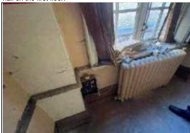
Photo 41 - Further examples of fallen ornamental plasterwork from the ceiling of the small hall.
