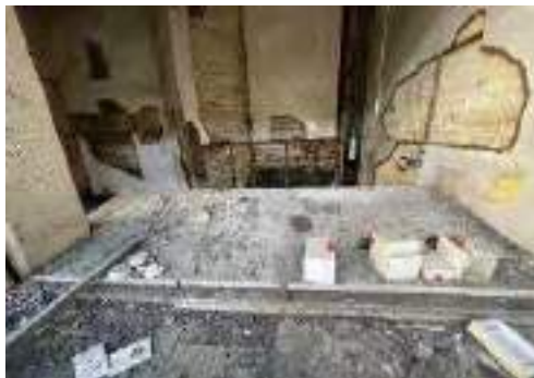
Photo 16 - Aged and defective finishes to the plastered walls of the units.
