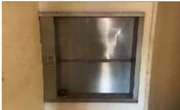
Photo 14 - Redundant dumbwaiter (1 of 2)
