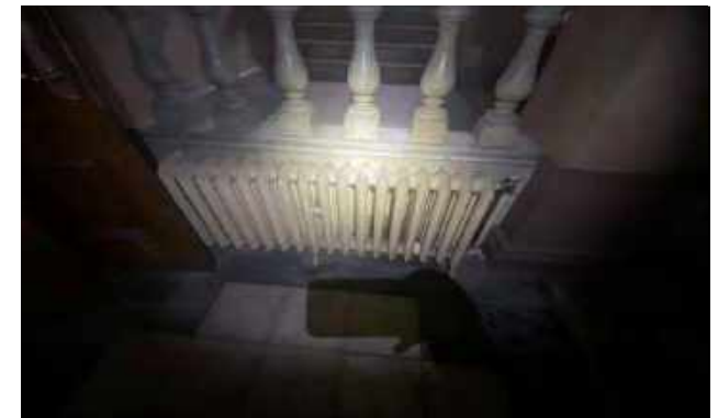
Photo 12 - Typical lobby area steel column radiator
