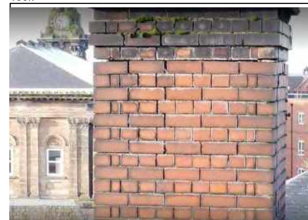
Photo 90 - Large chimney stack to South East displaying open joints and potential instability.
