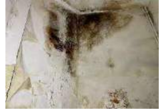
Photo 15 - Mould to the ceiling and walls of the toilets.
