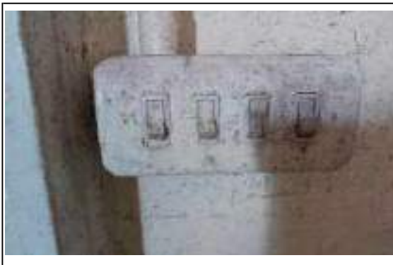
Photo 40 - Light switch that has been painted over
