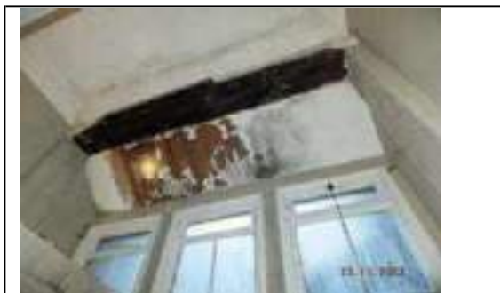
Photo 13 - Active water ingress to RG.19, timber saturated.
