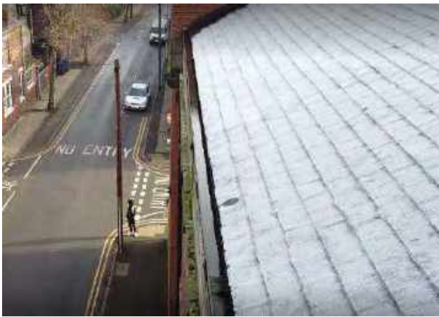
Photo 83 - Example trough gutter showing standing water (frozen).
