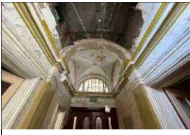
Photo 50 - Missing ceiling to the ground floor corridor area.
