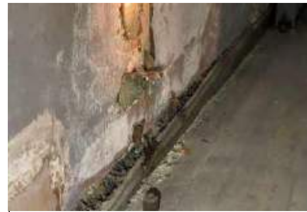
Photo 30 - Dry rot to the timber skirting board and wall above, in the gallery loft.
