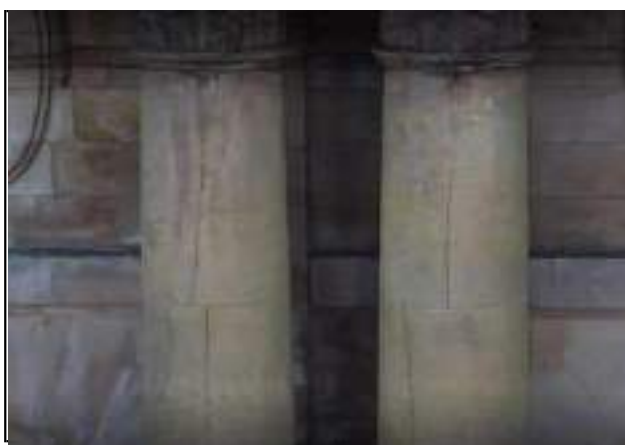
Photo 92 - cracking to stone columns on principal entrance.
