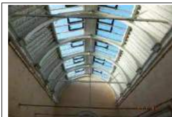
Photo 23 - Glazed rooflight over RF.23. Believed to have been repaired externally in 2017.
