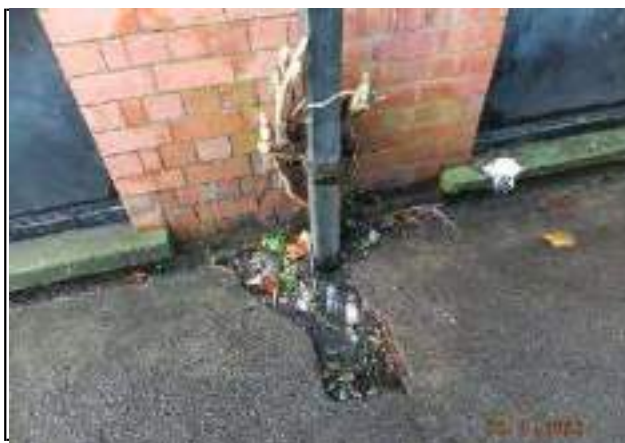
Photo 71 - Example damage to drainage surrounds.
