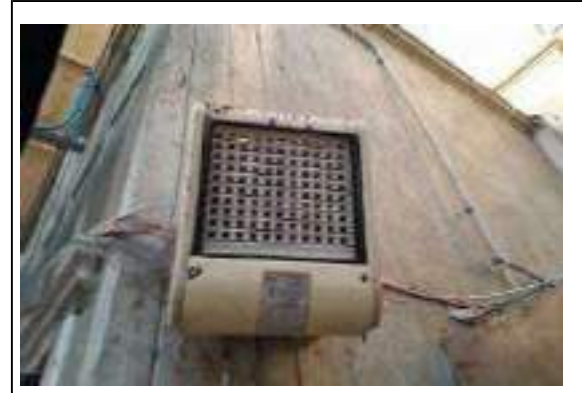
Photo 33 - Radiant plaque gas heater, disconnected from gas supply
