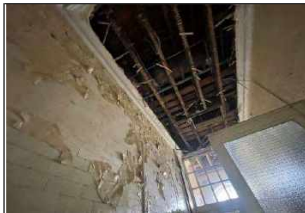
Photo 32 - Example of defective plaster throughout.
