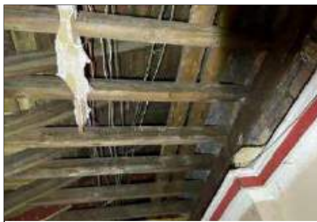
Photo 44 - Exposed timber trusses of the first floor corridor.
