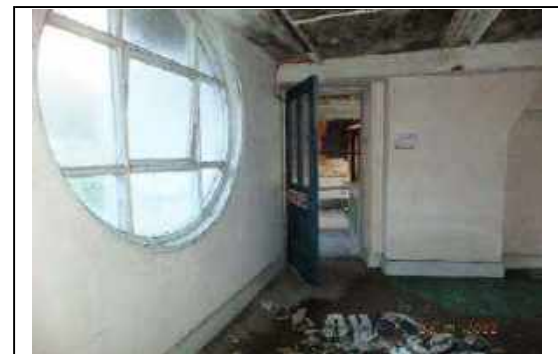
Photo 18 - View through RF37 (no further access). Collapsed lath & plaster ceiling and damage to floor below.
