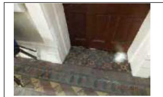
Photo 12 - Dry rot fruiting body emerging from RG.19 into RG.15
