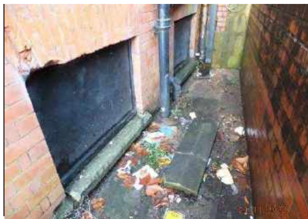
Photo 62 - Windows to basement (behind freestanding wall on Price Street). Damage to flat arch brickwork and missing coping stone.
