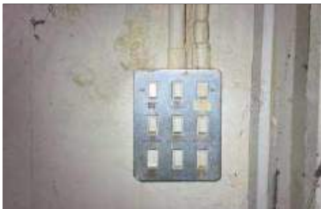
Photo 4 - Multi-gang lightswitch - typical dated construction and finish
