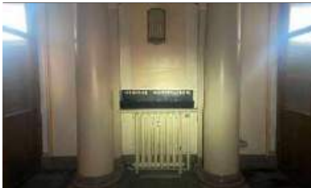
Photo 13 - Typical lobby area steel column radiator
