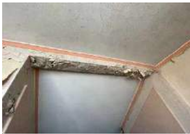
Photo 32 - Example of defective plaster throughout.
