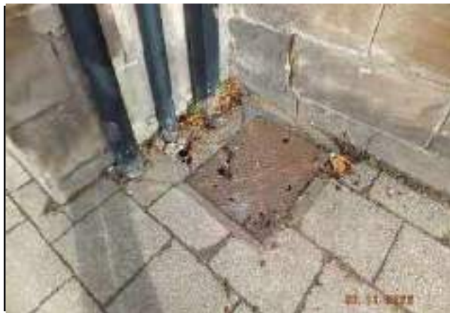
Photo 67 - Damaged manhole to Wedgwood Street.
