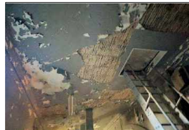
Photo 27 - View of roof access ladder and dilapidated ceiling within lighting control gallery
