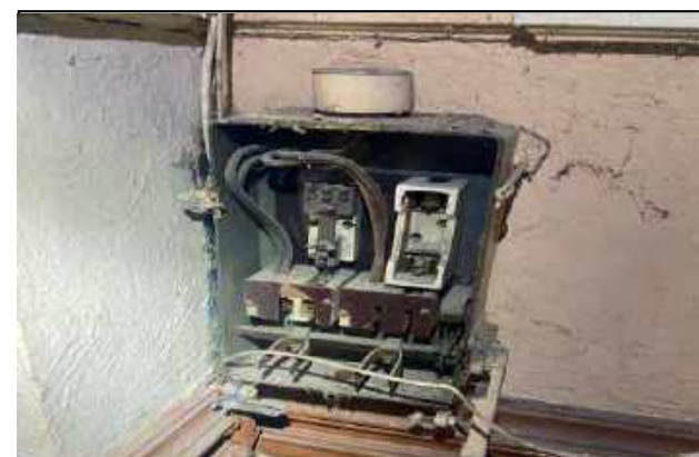
Photo 18 - Existing fusegear
