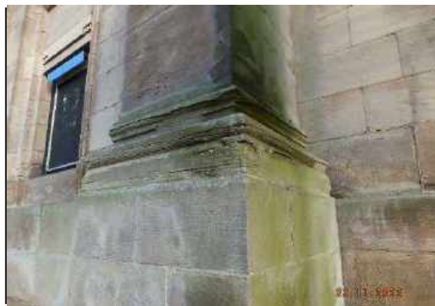
Photo 64 - Algae growth and deterioration of stone due to inadequate water shedding above.
