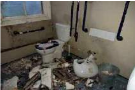
Photo 46 - Defective sanitaryware
