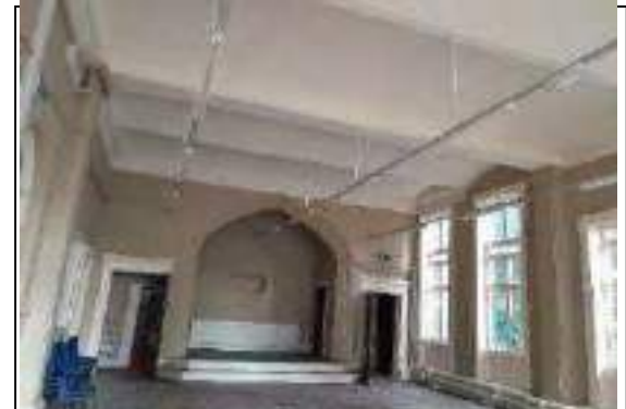
Photo 48 - Fluorescent luminaires with trunking wiring containment
