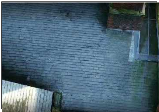
Photo 82 - Slipped slates to Princes Hall Western roof pitch along Price St.
