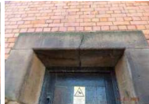
Photo 60 - Cracked lintel to stage entrance door.
