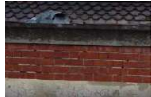
Photo 48 - Repointing needed to the front elevation.
