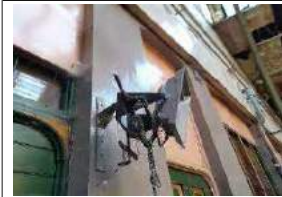
Photo 32 - Radiant plaque gas heater, disconnected from gas supply.
