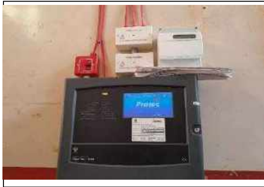
Photo 25 - Fire Alarm Panel
