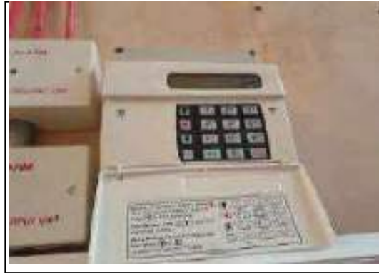
Photo 26 - Intruder Alarm Keypad
