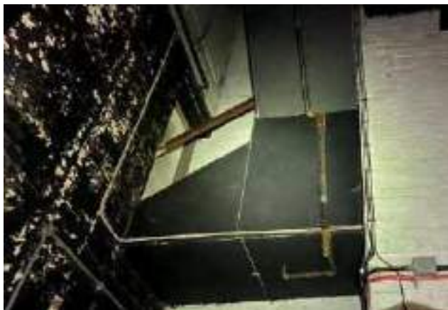
Photo 25 - Corroded sprinkler system pipework in stage area
