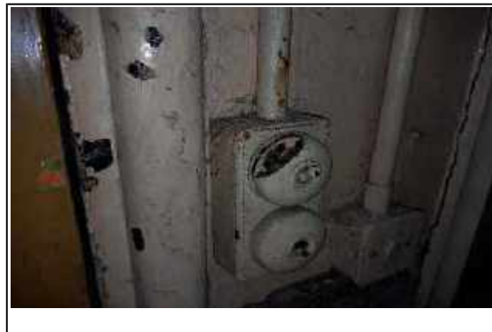
Photo 41 - Damaged period light switch
