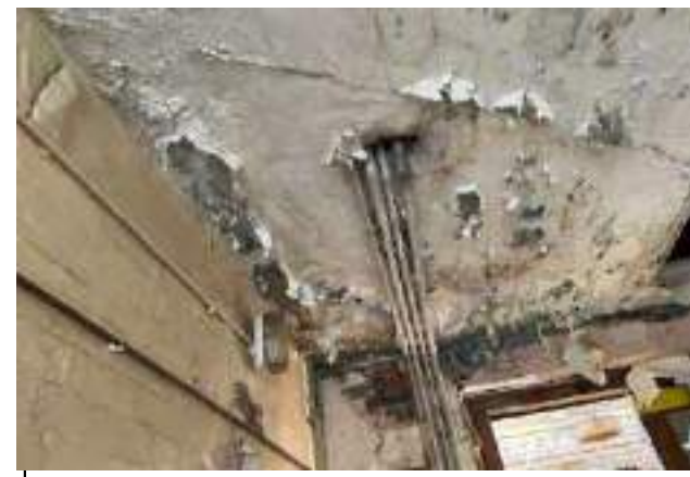
Photo 48 - Typical water damaged ceiling
