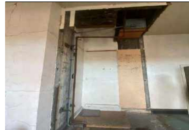
Photo 21 - Redundant water storage/F&E tank with corroded pipework
