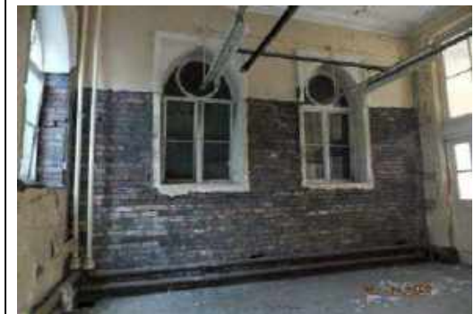
Photo 30 - View of 'external' wall & windows to North side of RF.26. Evidence of previous dry rot or waterproofing injection treatment to lightwell walls.
