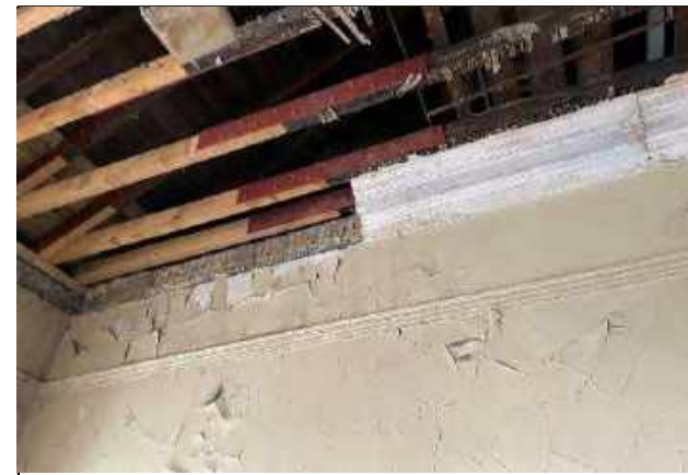
Photo 39 - Past example of splicing to the timber trusses within the roof voids of the first floor.
