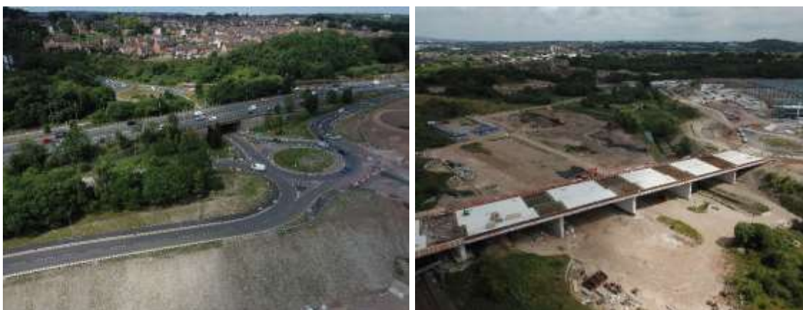
Images 15 & 16 - Etruria Valley Link Road Under Construction
