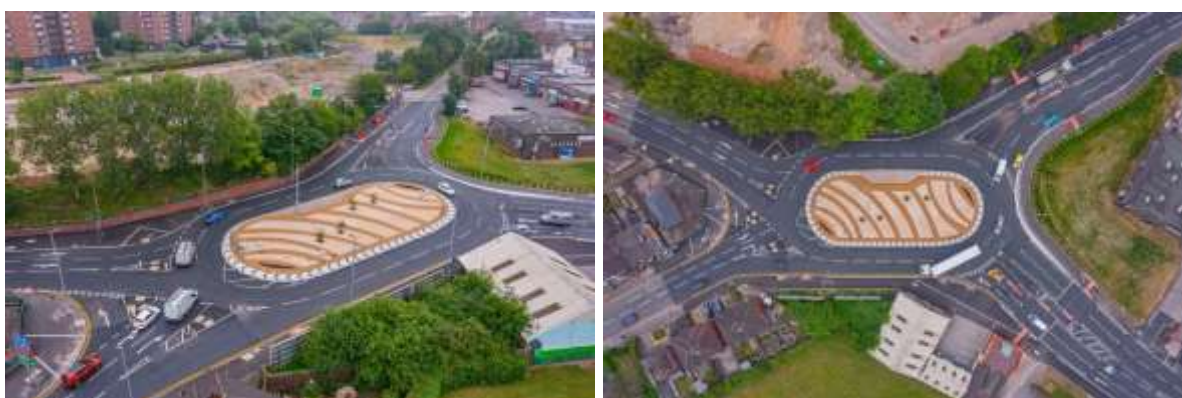
Images 13 & 14 - Joiners Square Roundabout Improvements
