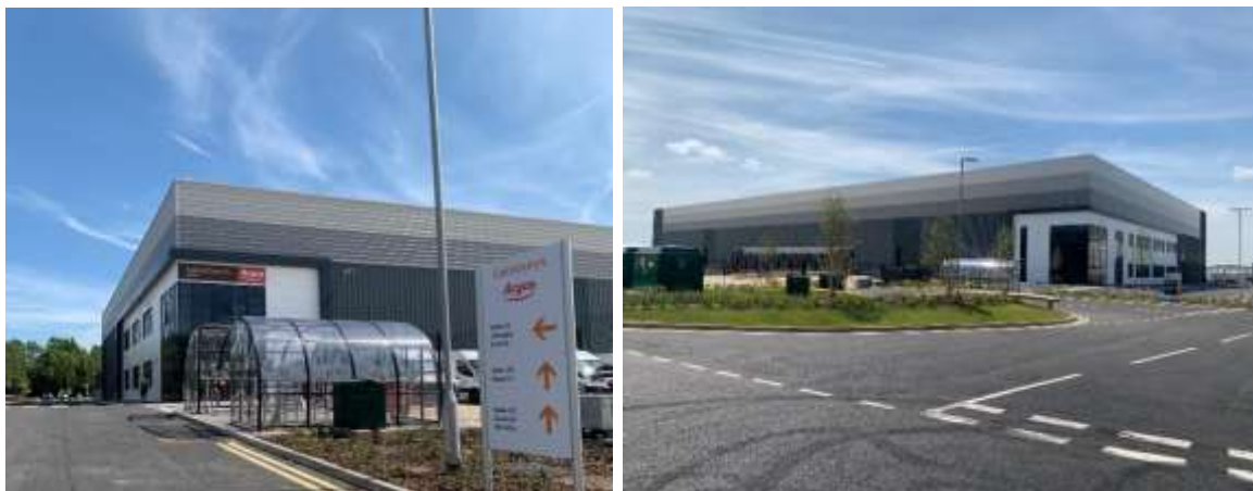
Images 9 & 10 - Distribution warehouses, Stoke, Gordon Banks Drive
