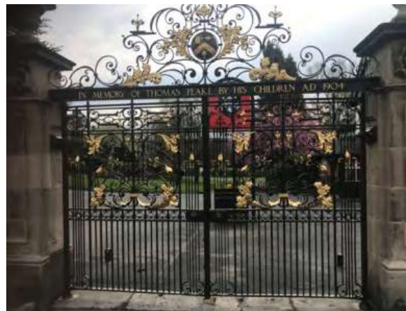
Images 22, 23 and 24 – Refurbishment works Tunstall Park - 106 monies used from application 40915/FUL
