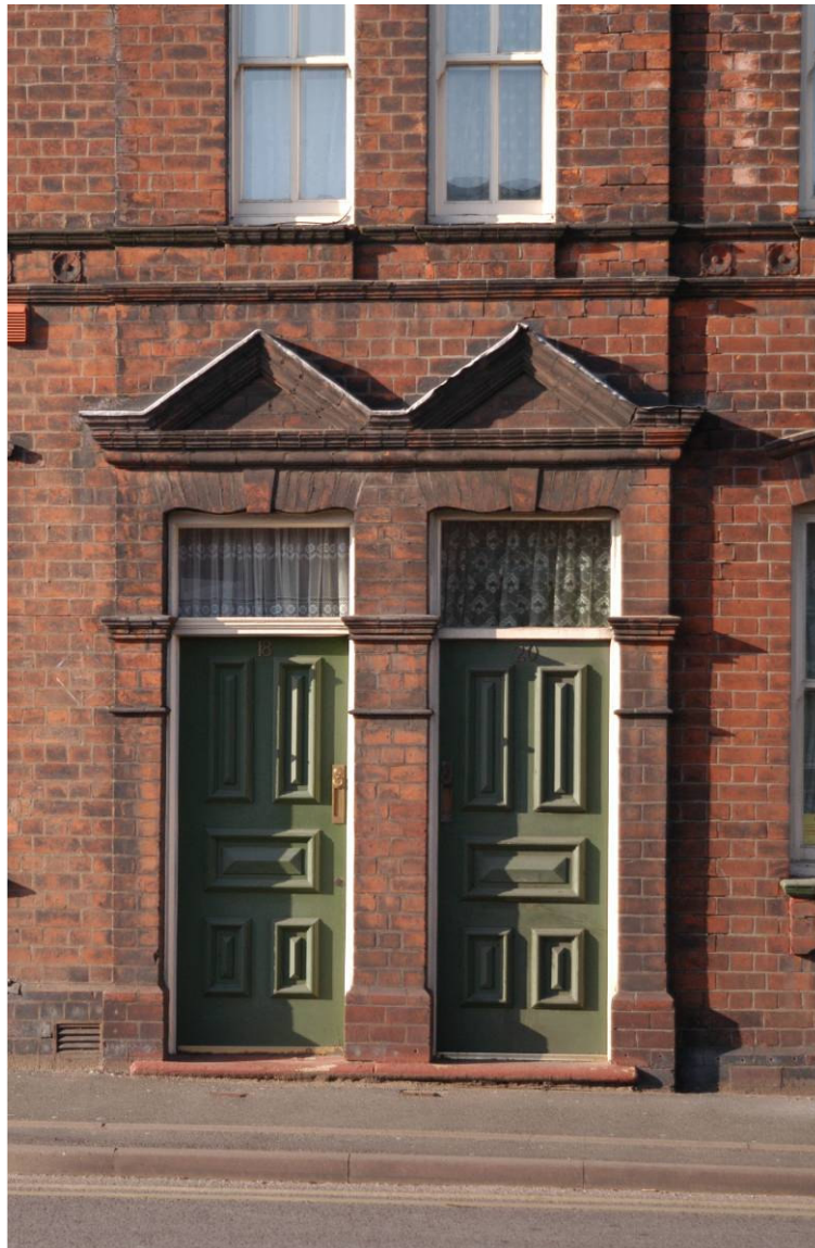
FIGURE 14: Doors with the simplest brick door-case.
