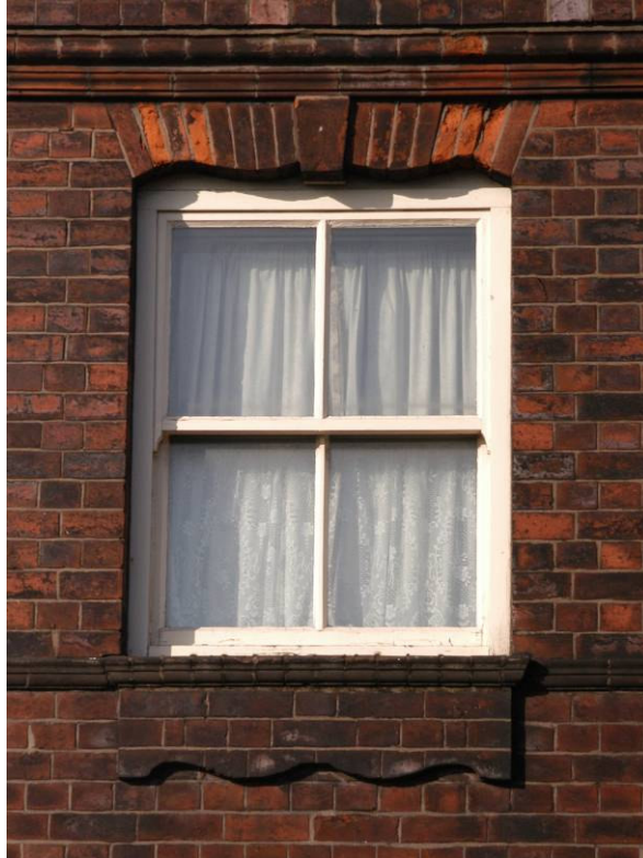
Figure 13: Windows with moulded aprons and curved arches
