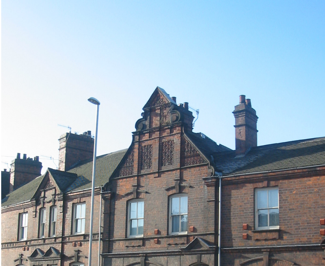
FIGURE 12: Roofs, chimneys and original moulded chimney pots
