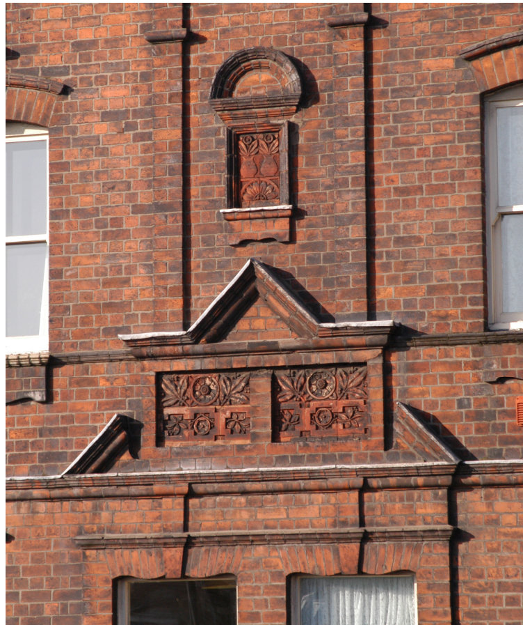
FIGURE 15: Detail from larger door-case showing decorative brickwork over door fanlights
