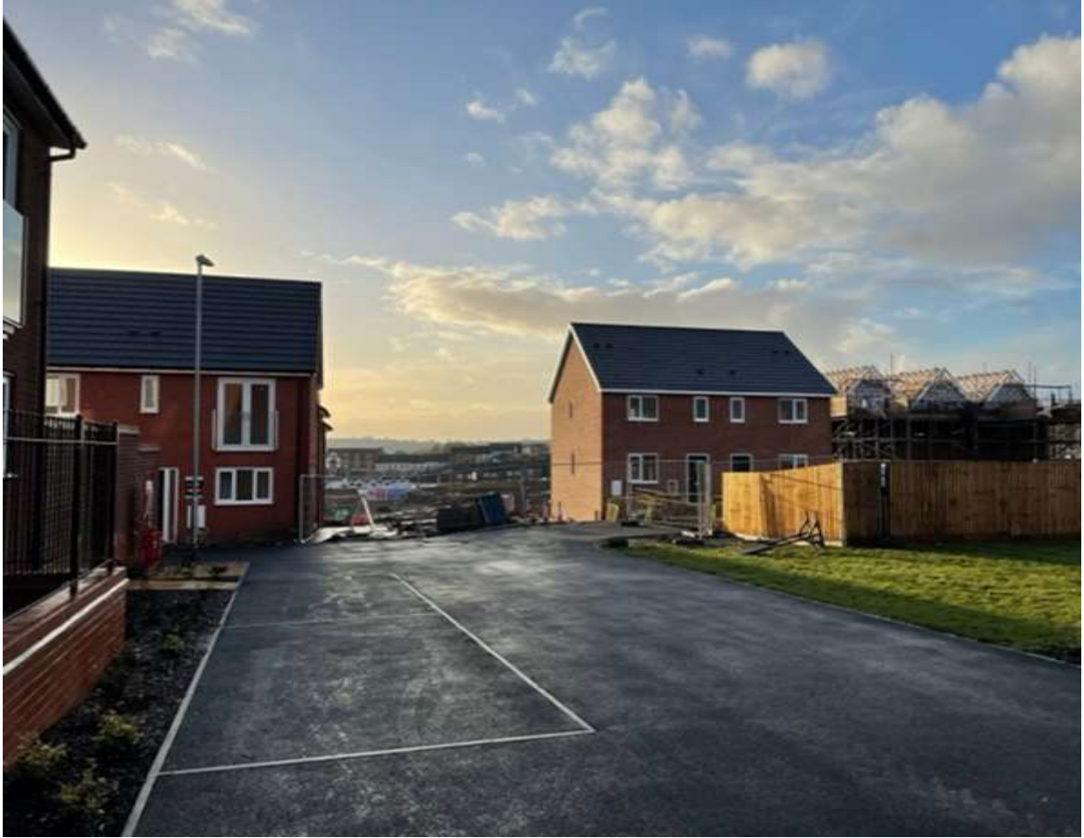
Former Royal Doulton Site, Burslem (63695) – Under Construction
