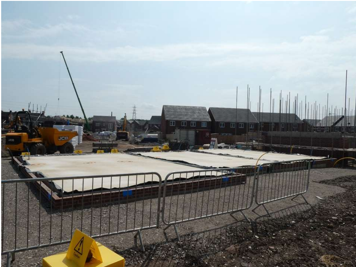
Victoria Ground site 61254 – Under Construction
