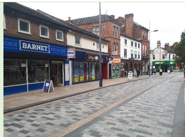
Figure 2: Recent investment in the public realm within Hanley has had an overall positive effect on the city centre.
