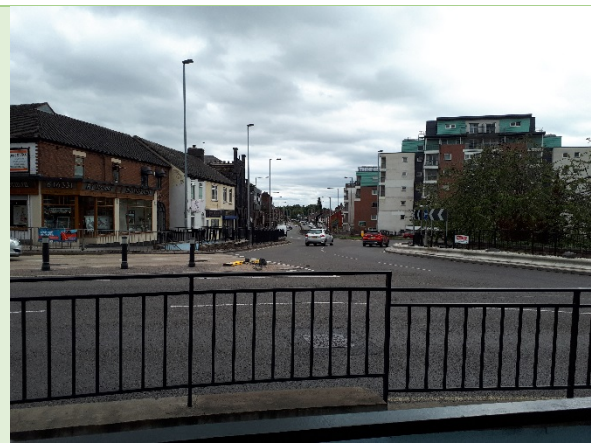
Figure 2: The centre is surrounded at all sides by a dual carriageway, which impedes movement
