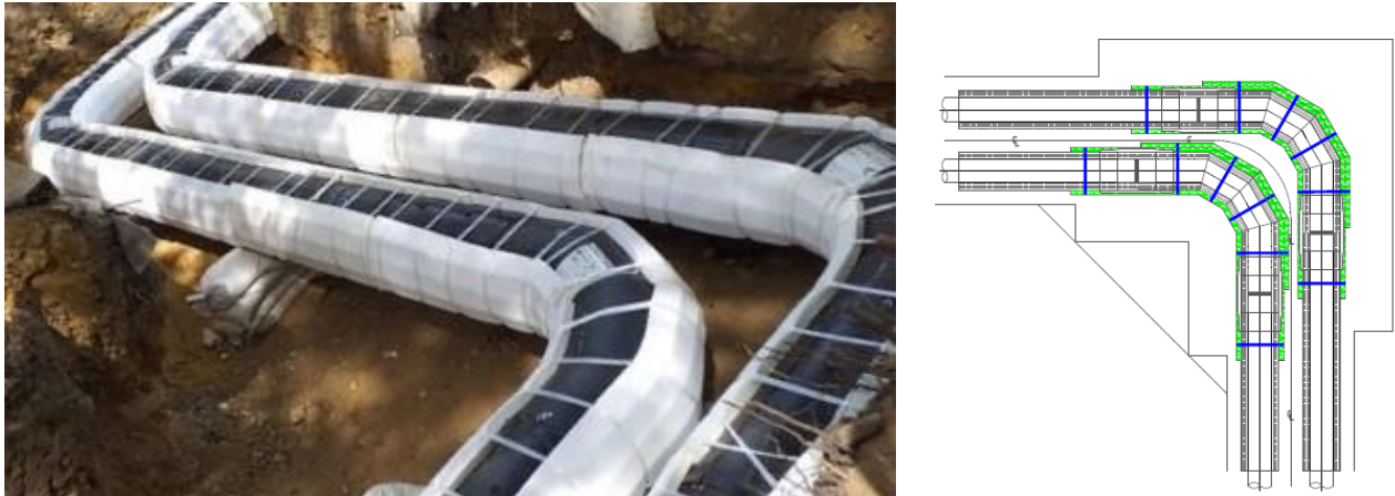
Figure 14 - Typical Expansion Cushion Arrangement.
