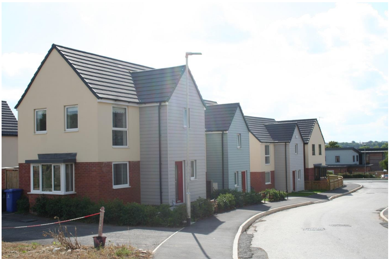
Bucknall Former Hospital 58877 – Under Construction
