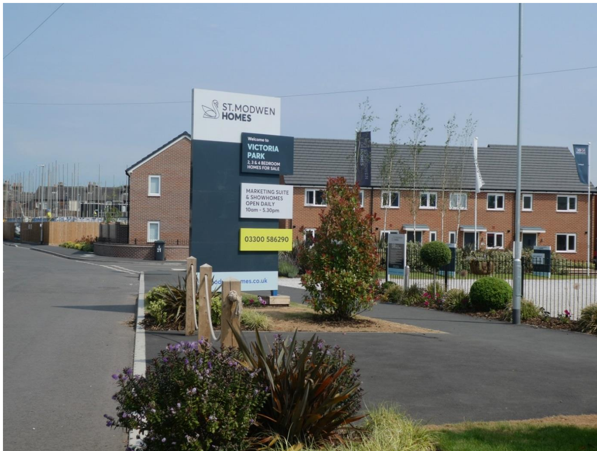
Victoria Ground site 61254 – Under Construction
