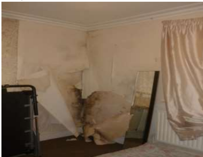
Damp and mould
