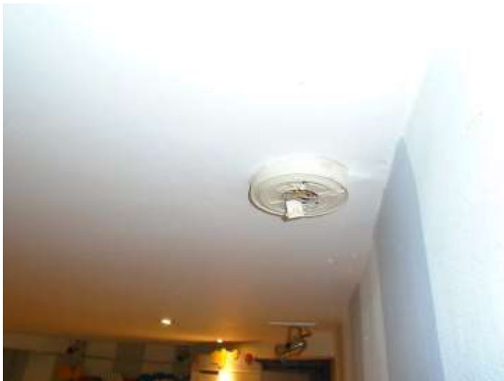
Non working smoke detection
