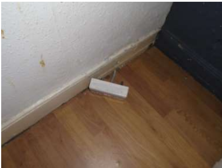
Non working smoke detection
