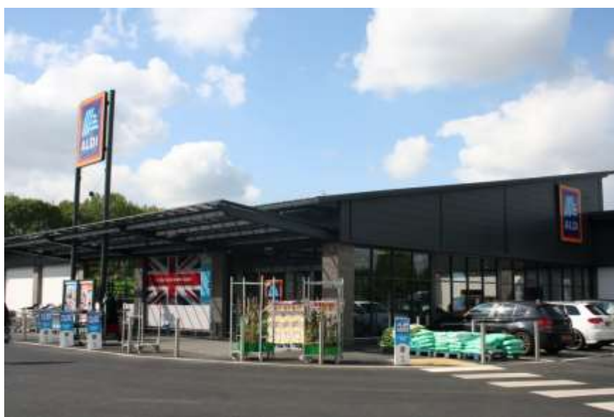
ALDI Stores Ltd, Whittle Road, Meir (61298) – Complete
