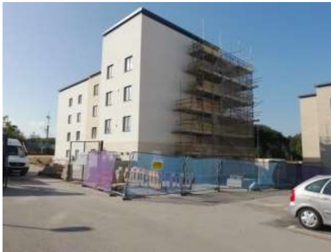
Premier Inn (extension), Etruria Road (60782) – Under Construction
