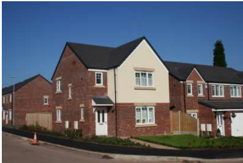
Dyson Ceramic Systems, Shelton New Road (60831) – Under Construction
