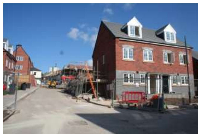
City Centre Waterside, Hanley (58689) – Under Construction
