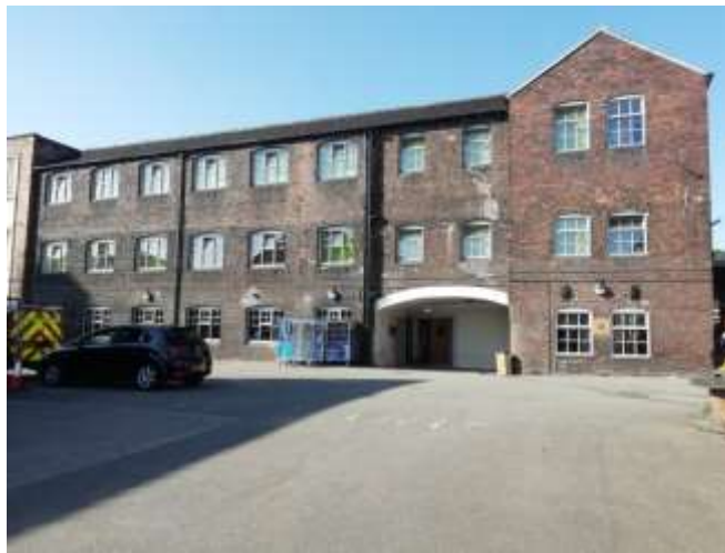
Potbank Aparthotel, Spode Works (61504) – Under Construction
