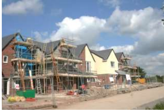
Former Bucknall Hospital, Eaves Lane (58877) – Under Construction
