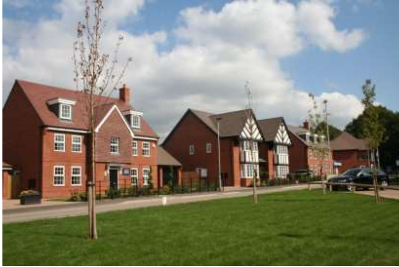
Wedgwood Development Site (The Oaks) (55286) – Under Construction
