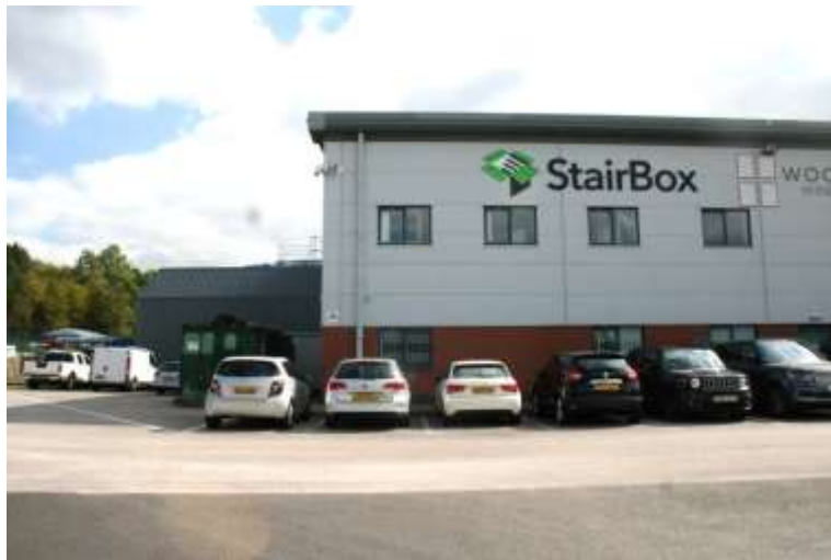
Stairbox, Gordon Banks Drive, Trentham Lakes (60179) – Complete
